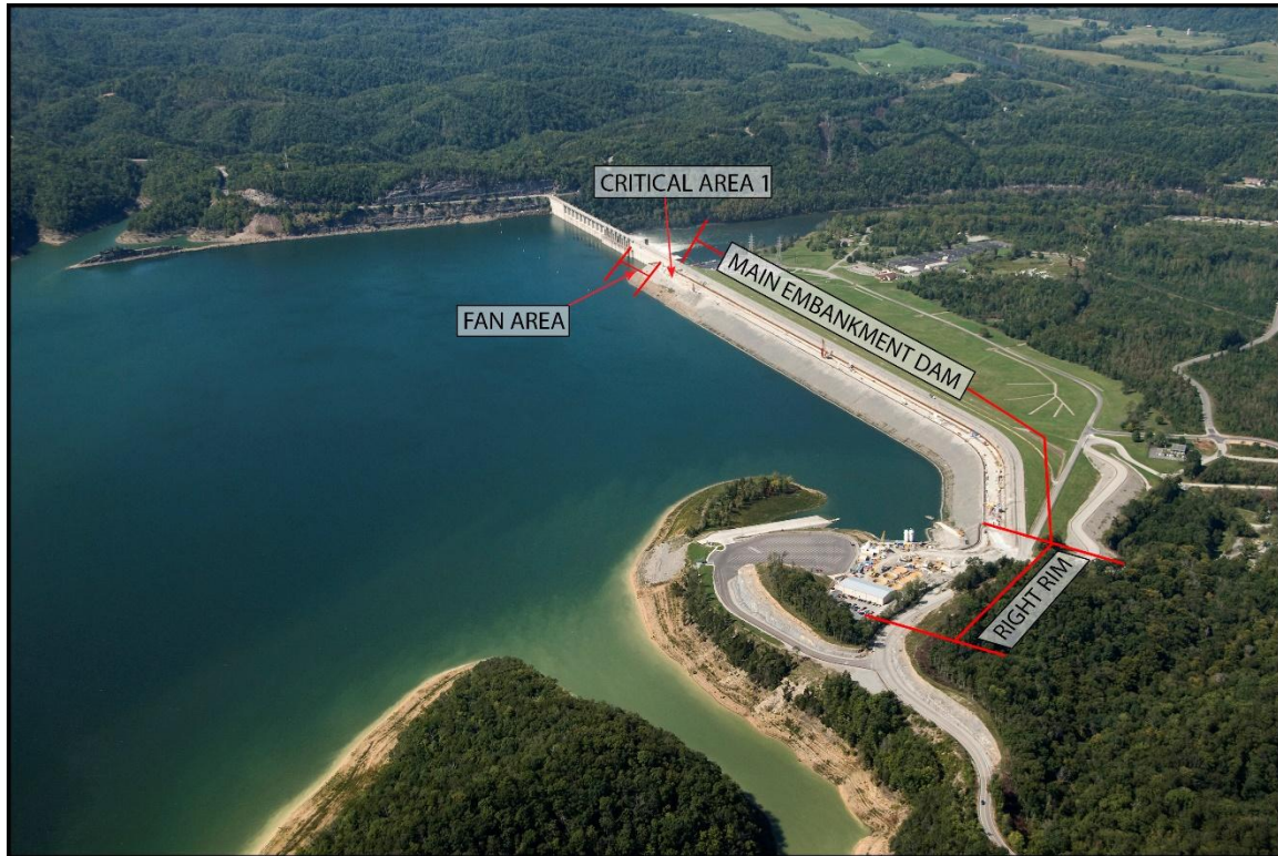
Figure 14. Wolf Creek Dam during construction in September 2009. TSJV Plant in foreground – HMG grouting program and barrier wall construction installation in background.
