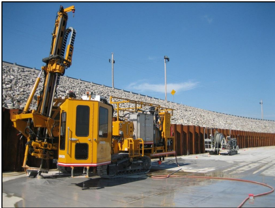
Figure 13. Crawler drill rig with Water-Powered Down-the-Hole (WDTH) Hammer.
