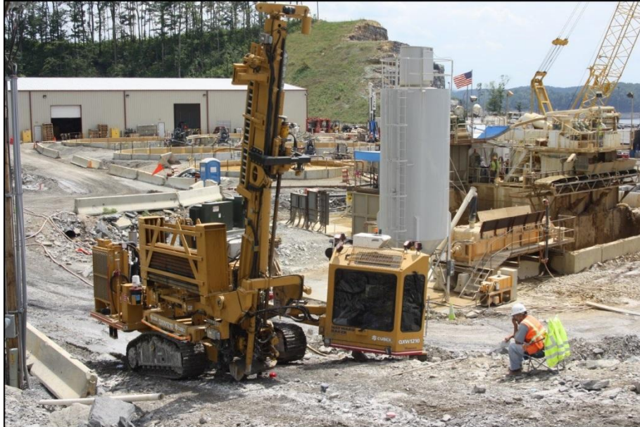
Figure 16. Right Rim - Rock drilling with TSJV cut-off wall slurry and desanding plant in background.
