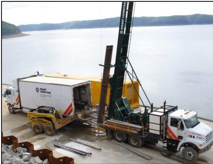
Figure 12: Truck mounted Sonic Drill.
