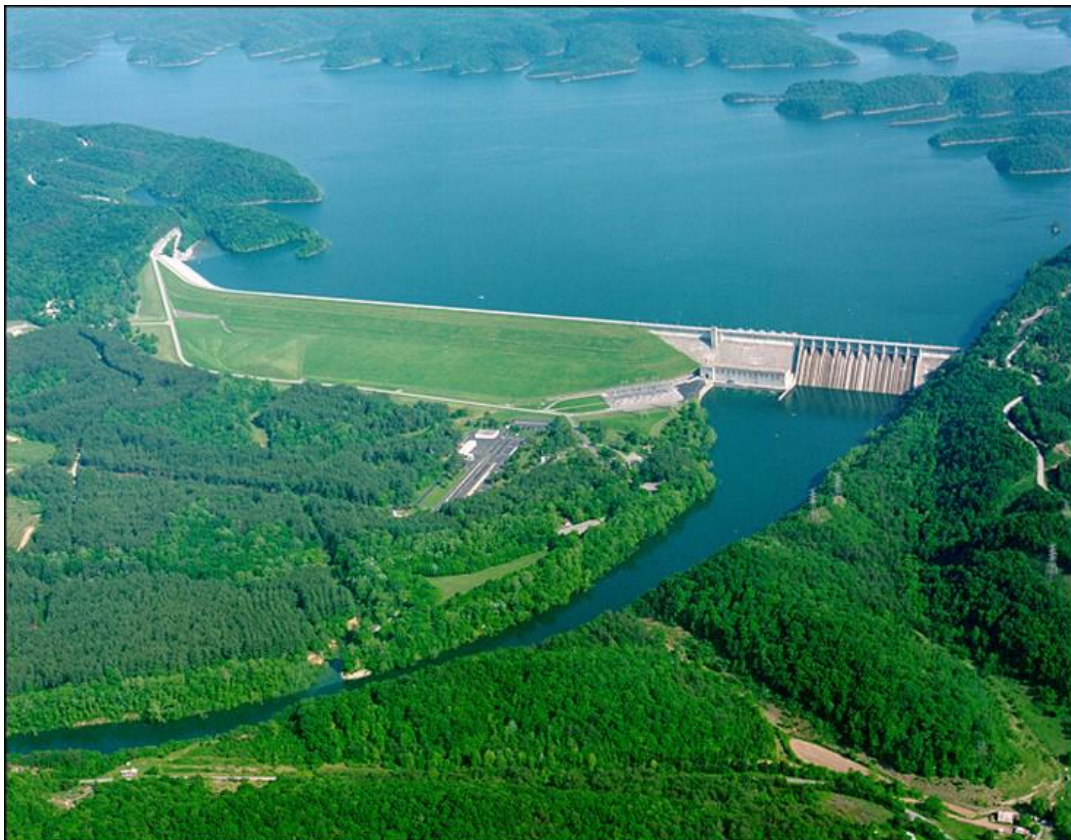
Figure 2. Aerial View of Wolf Creek Dam showing the concrete gravity section (including powerhouse) on the Left Abutment and the embankment section to its right (Source: USACE).
